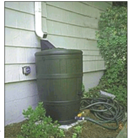
A rain barrel used to collect rooftop runoff using a gutter / downspout system
