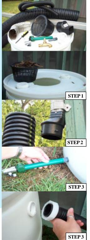
٨ Overflow connector and drain hose
