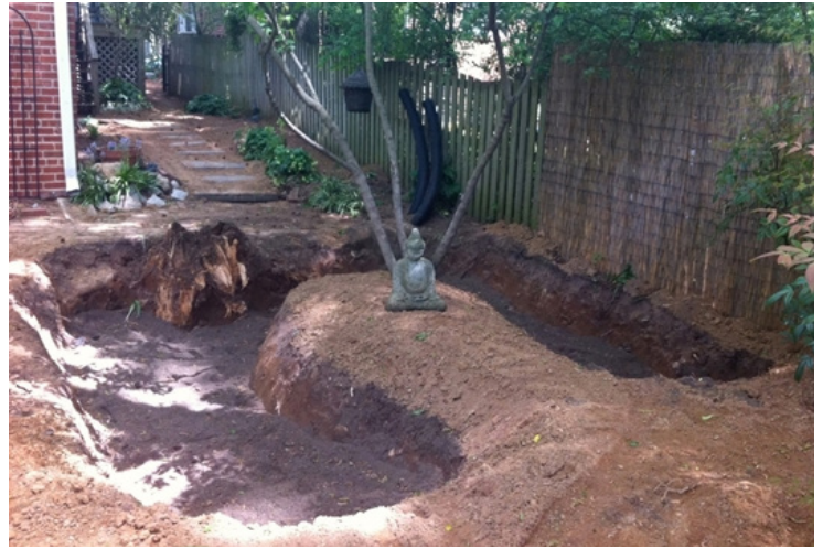
Figure 5.5-2. BMP Initial Verification Visual Indicators Present: 2, 3, and 11
