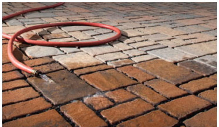
Figure 5.4-3. BMP Initial Verification Visual Indicator Present: 7
