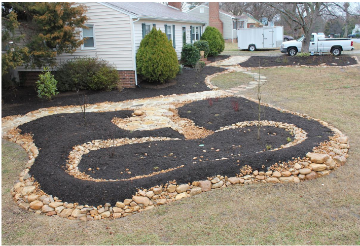
Figure 5.5-3. BMP Initial Verification Visual Indicators Present: 1, 3, 4, 5, 7, 8, 9, and 10
