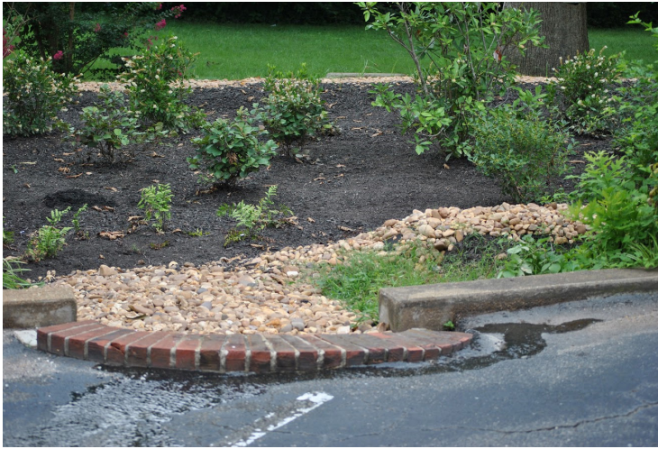
Figure 5.5-1. BMP Initial Verification Visual Indicator Present: 9
