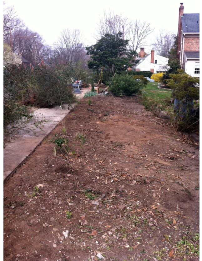
Figure 5.7.b. BMP Performance Verification Visual Indicators Present: 1, 3, 4, 5, and 6
