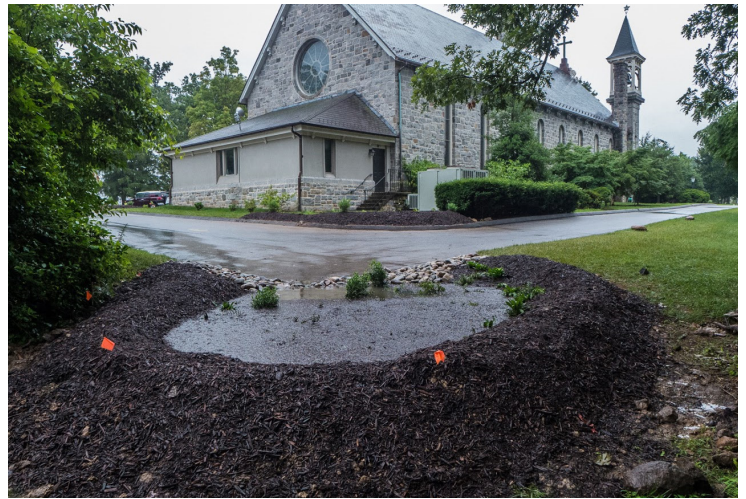
Figure 5.5-4. BMP Initial Verification Visual Indicator Present: 14
